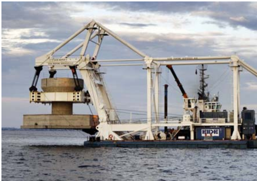
Figure 6: The crane places the foundation in its exact position
