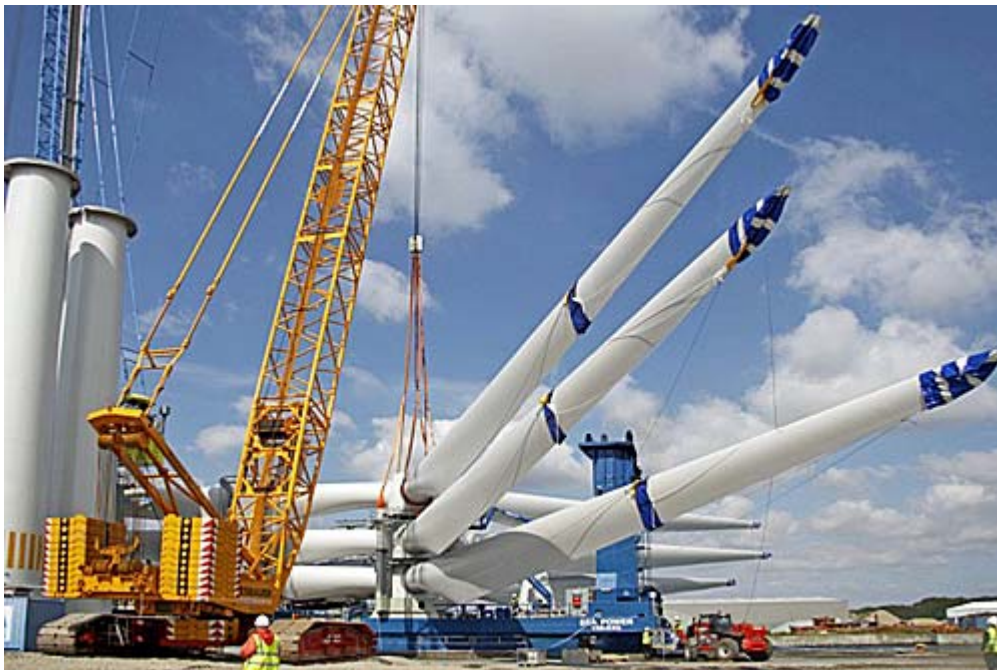
Figure 6: Loading the wind turbines in the harbour
