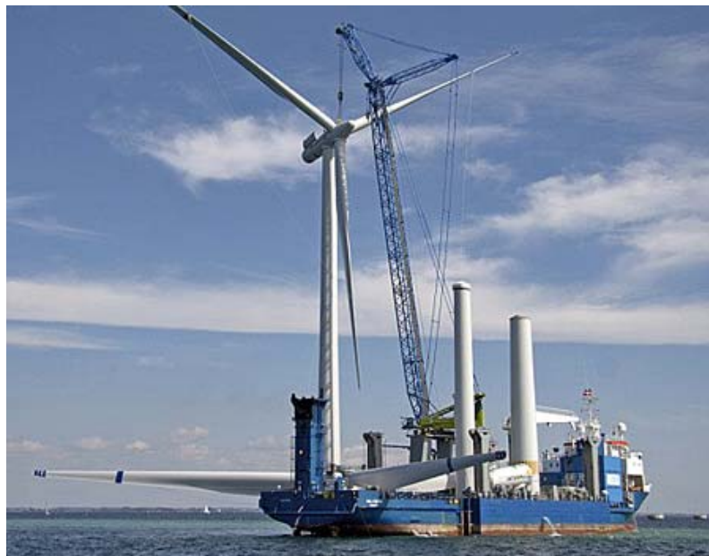
Figure 8: Wind turbine installation
