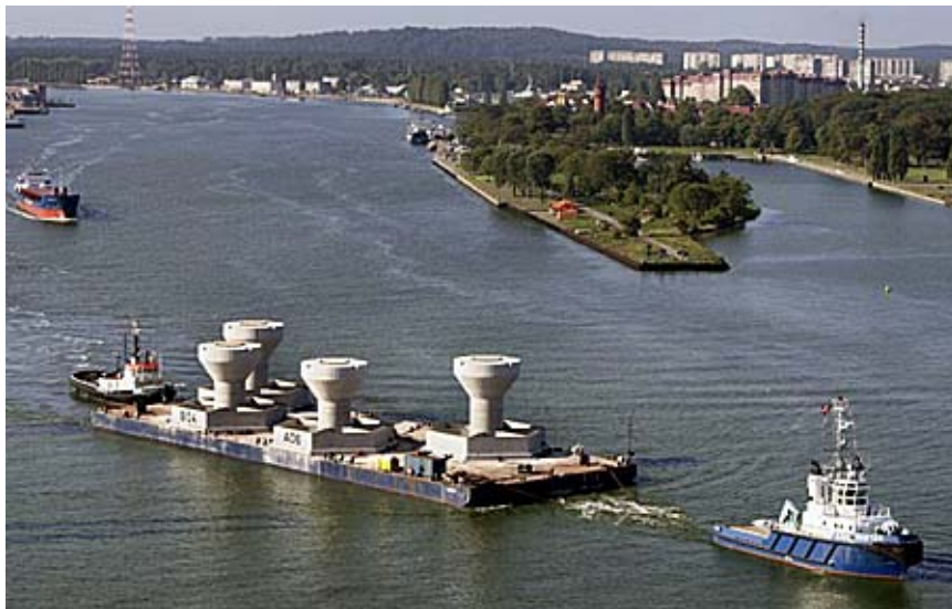
Figure 5: A tug takes the barge with four foundations from Poland to Lillgrund
